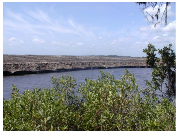
Levee Reach J-1 Construction
